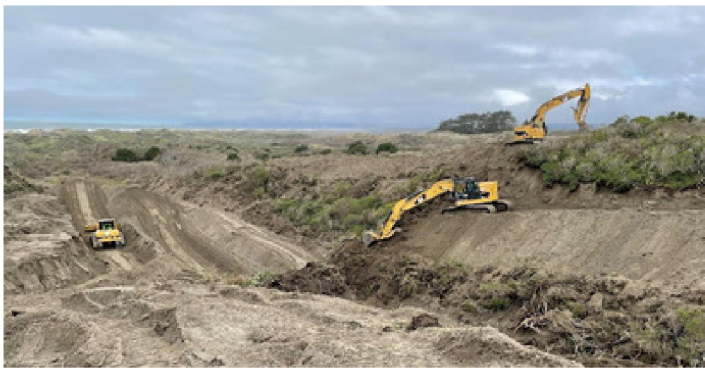
Heavy equipment operated by GR Sundberg scraping the lupine/duff layer and burying it in trenches at the Wadulh Unit of the Humboldt Bay National Wildlife Refuge. Photo by Andrea Pickart.
